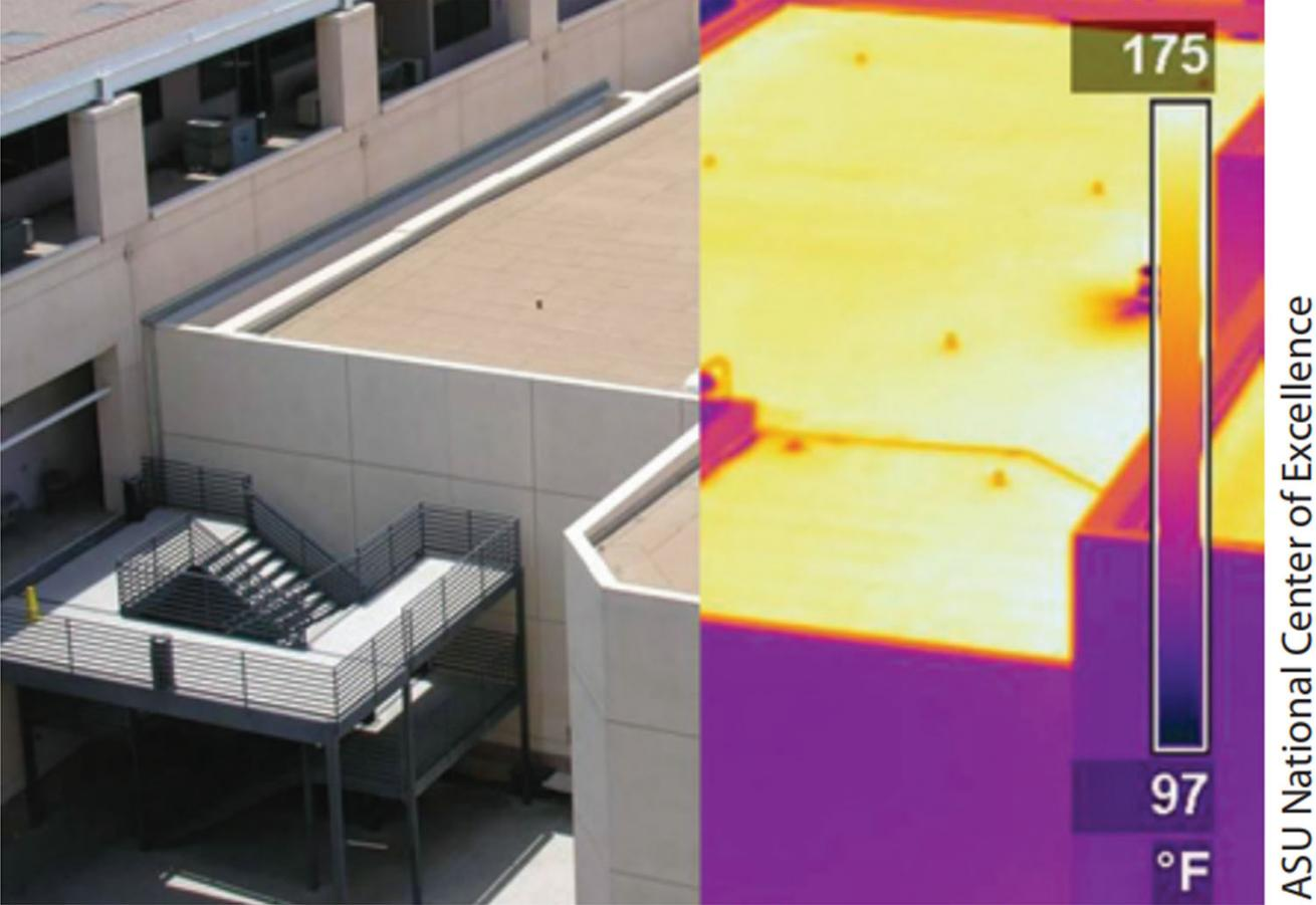
Temperature of Conventional Roof reached 175degF (80degC)
